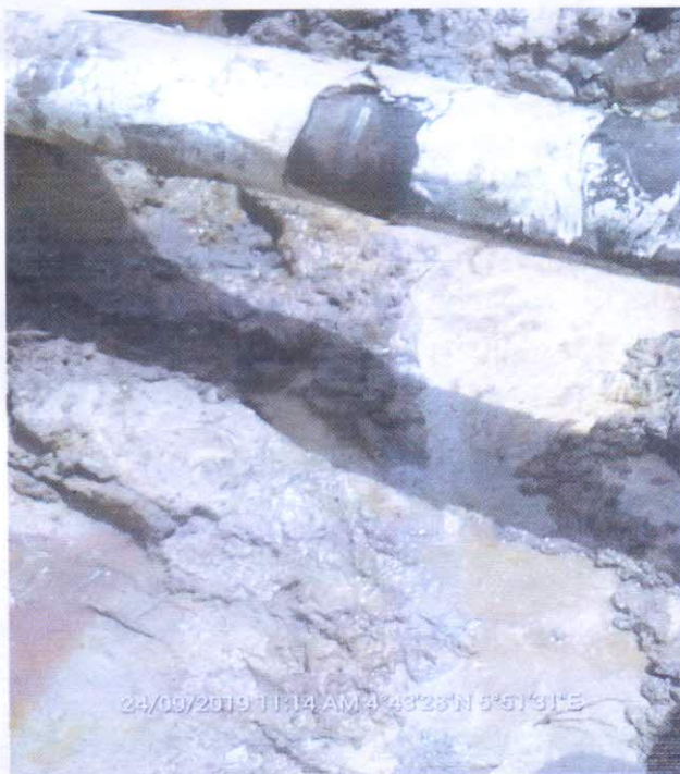
THE POINT WAS WELDED.
