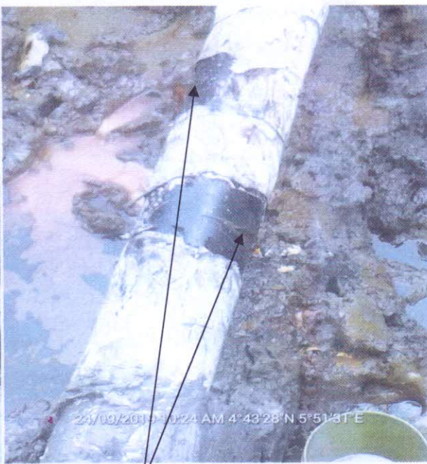
HACKSAW CUT AT TWO DIFFERENT POINTS.
